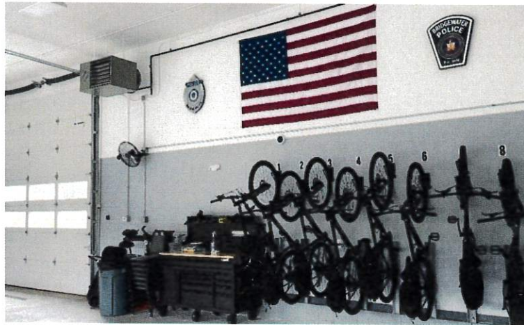
Outbuilding garage bay area
