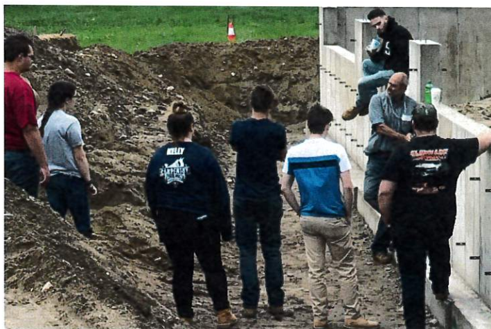
Outbuilding construction started in 2019 by B-P students and supervised by Carpentry Instructor Doug Coray
