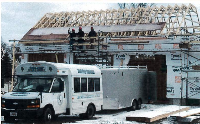
Outbuilding roof installation
